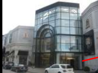
Atrium Mall, Boston
